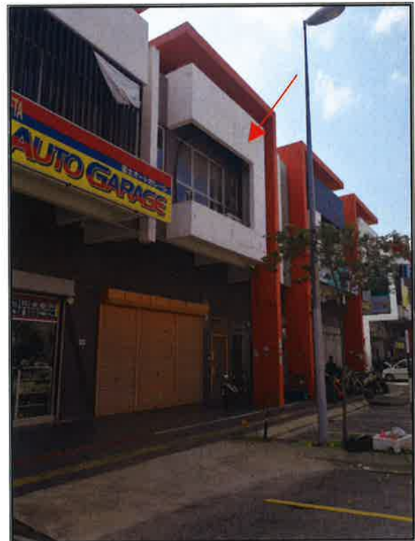
General view of the Property (indicated by a red arrow) in relation to its surrounding.
