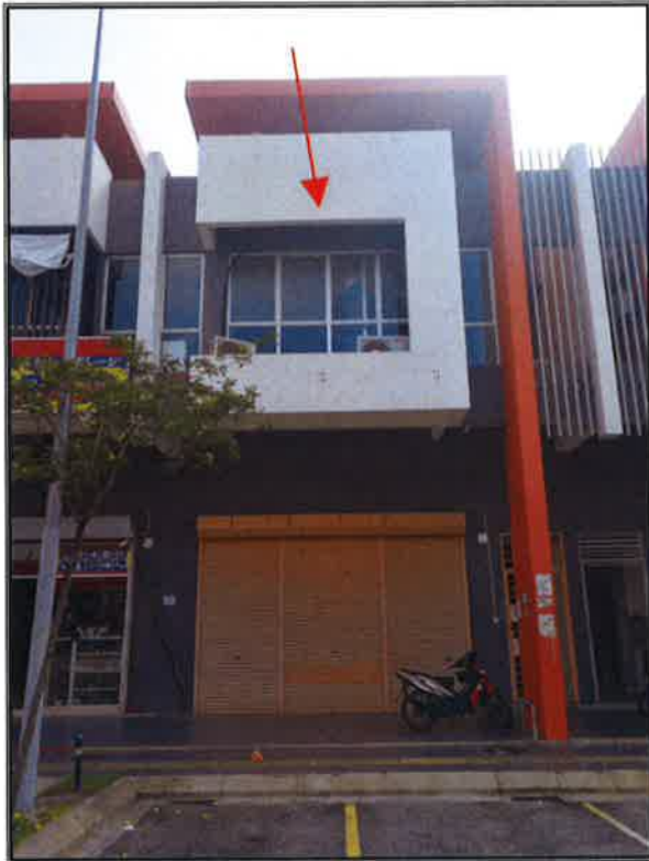
Front view of the Property (indicated by a red arrow)
