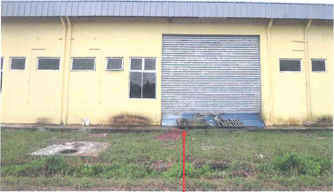
REAR VIEW OF THE BUILDING
