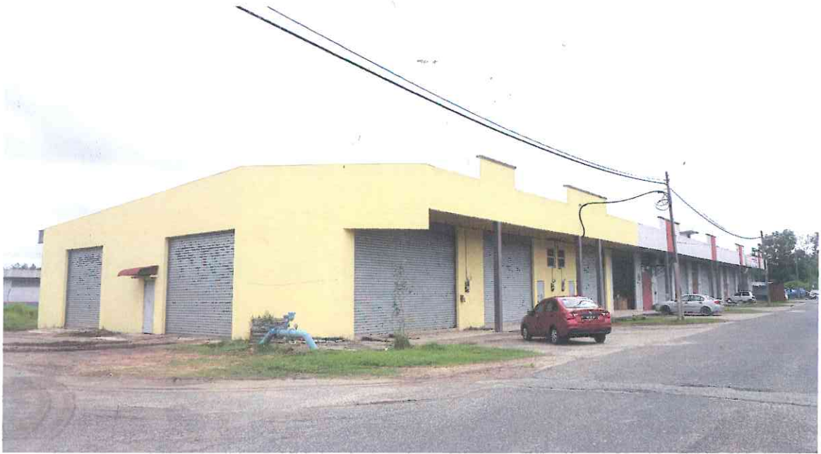
GENERAL VIEW OF A ROW OF SINGLE STOREY TERRACED FACTORY
