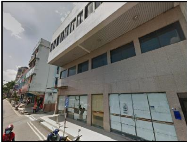
Left View of Subject Property
